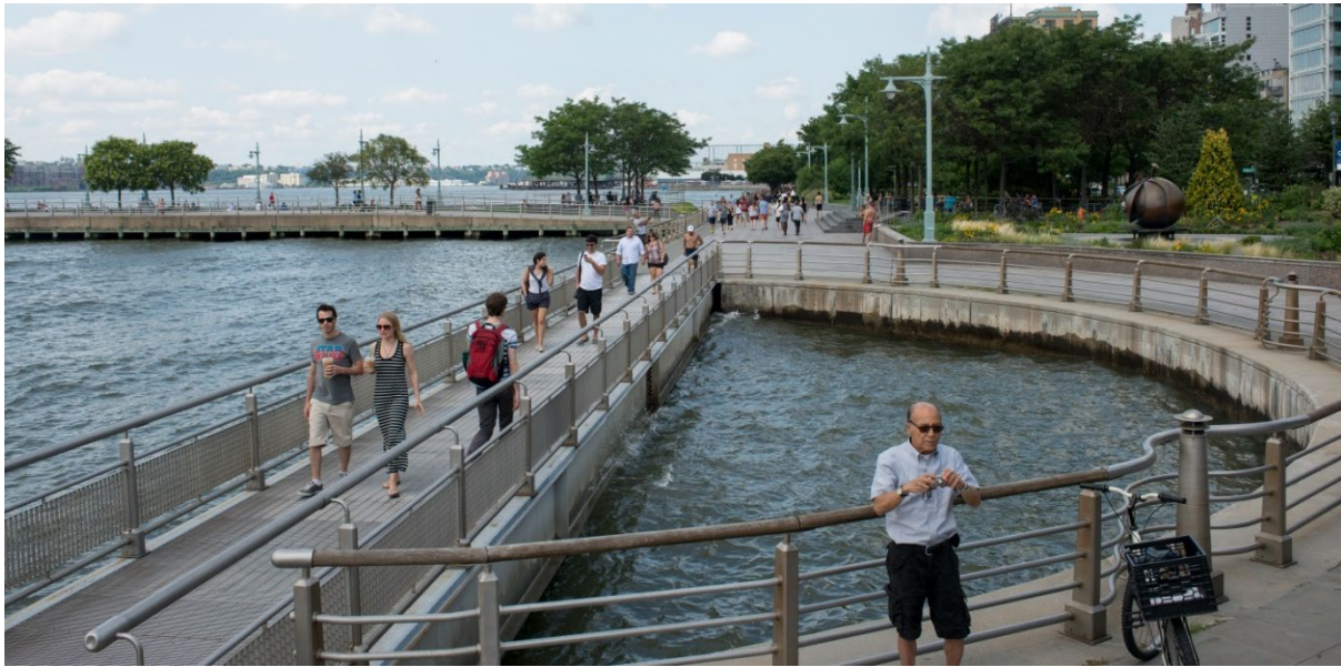
Figure 24: A bow notch located on the esplanade between Piers 45 and 46 in the West Village highlights an era of maritime history when, during the early twentieth century, port operators cut out notches from the existing seawall to accommodate larger and longer vessels.
