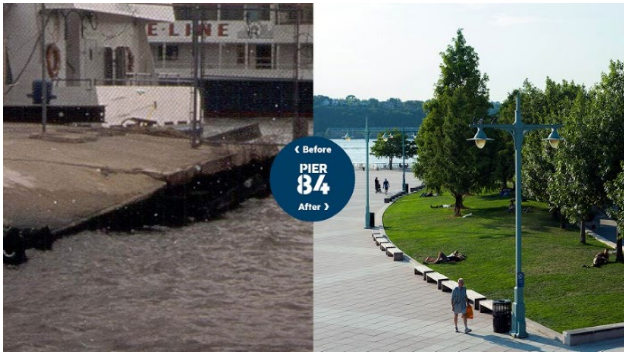
Figure 19: Rebuilt in 2006, Pier 84 stretches almost 1,000 feet into the River and measures nearly 100,000 square feet, making it one of the largest piers on the Manhattan waterfront.
