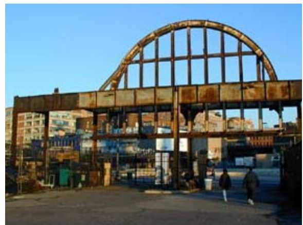
Figure 23: This steel archway from the former Pier 54 headhouse was left in place when the building was removed prior to the Park’s construction and was recently preserved as an icon of the bygone oceanliner era.
