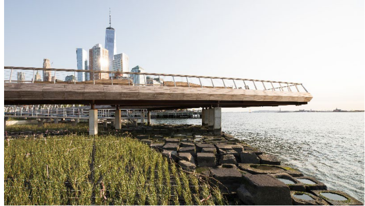
Figure 41: The Tide Deck, located at the western end of Pier 26, is an engineered rocky tidal marsh created to provide an immersive and educational river ecology experience for students and Park visitors.
