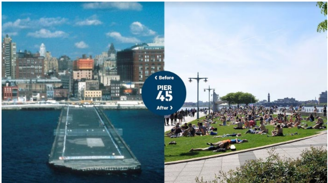
Figure 15: Completed in 2003, Pier 45 was one of the first piers to be rebuilt by the Trust and is a treasured asset for the West Village community and beyond.
