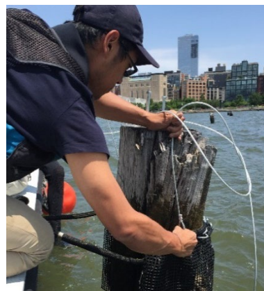
Figure 62: River Project staff installs an oyster wrap at Pier 32.
