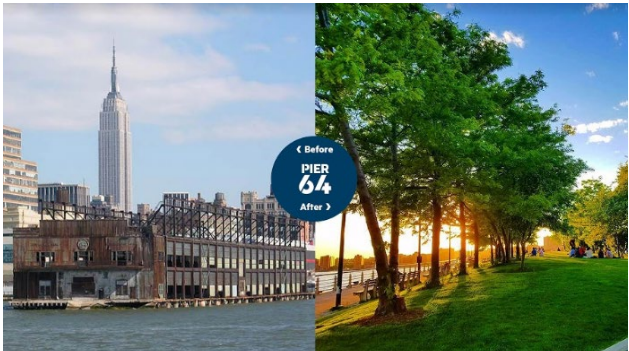
Figure 17: An area once filled with deteriorating steel beams is now lined with tall trees and shaded lawns. Pier 64 in Chelsea is part of the largest contiguous green area in the Park.
