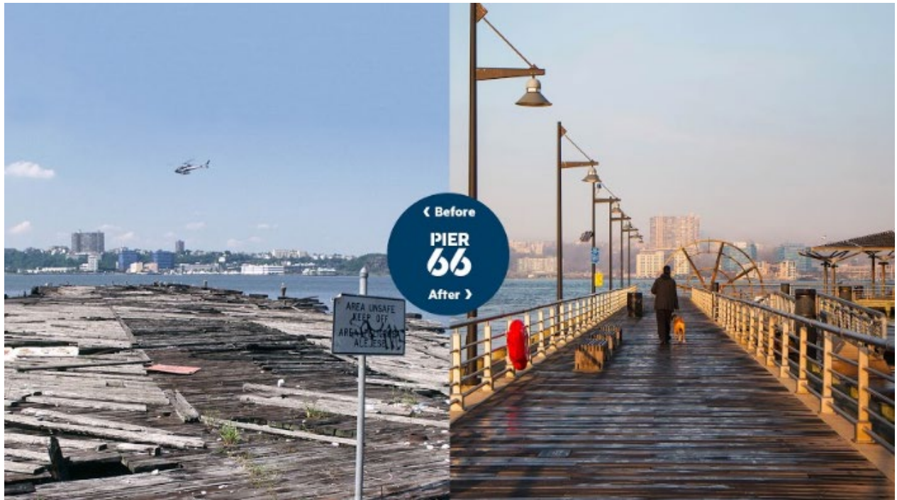
Figure 18: Pier 66, an area once condemned as unsafe, is now a public pier featuring a non-motorized boathouse and Long Time by Paul Ramires-Jonas—a water wheel sculpture that captures the beauty of the Hudson River while harkening back to its shipping and milling history.
